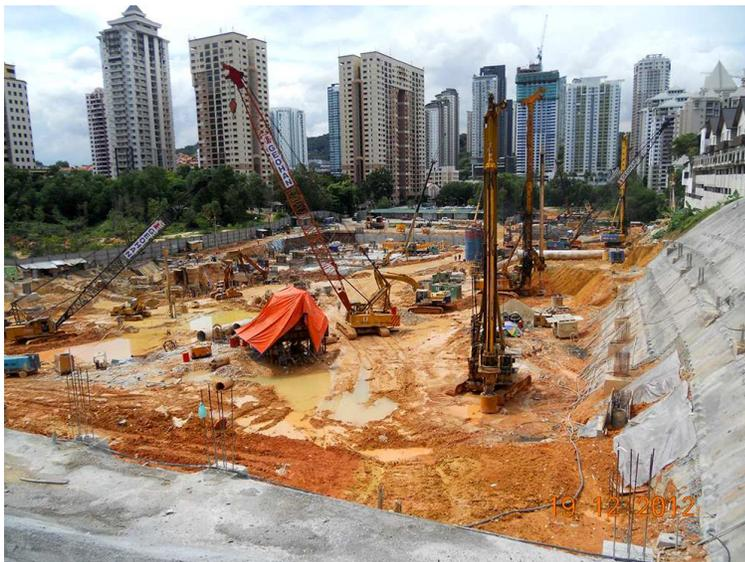
Based on the subsurface investigation (SI) report, the geological profile of the site is granite residual formation with varies of bedrock level and inconsistency of weathering grade of Granite rock over the site. The pile is designed to be founded on rock socket or maximum fixed pile length if no rock was encountered. Due to the deep layer of overburden soil, the soil friction is taken into account for optimisation of rock socket length required.
