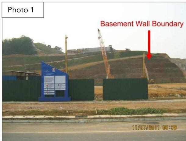
slope, the exposed cut surface was noticeably remains dry and consists of medium to stiff soil and highly weathered sandstone, with no groundwater was encountered.
